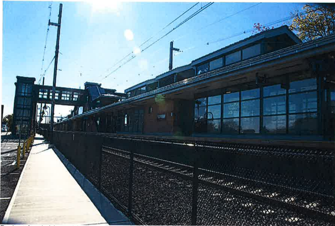
Pedestrian bridge with transparent materials – South Amboy, NJ
