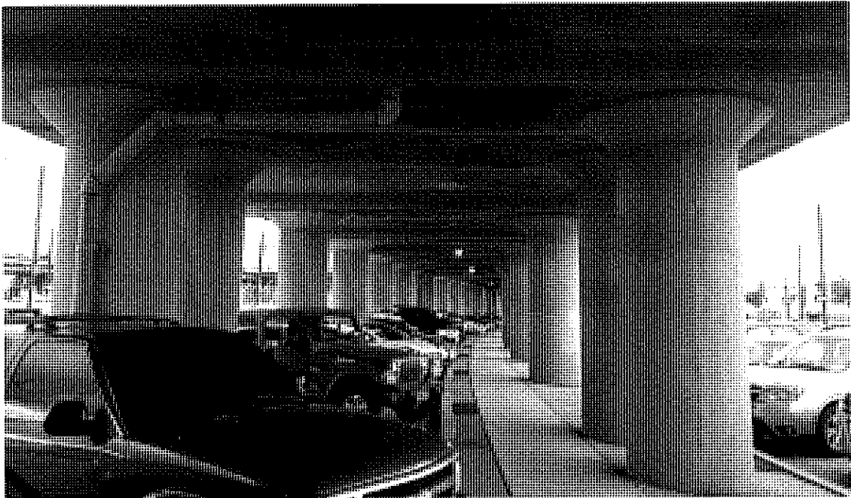
West-facing view of the LIRR overpass in the northeastern region of Lot H-11. No pigeon droppings observed where the base of the LIRR overpass is solid concrete.
