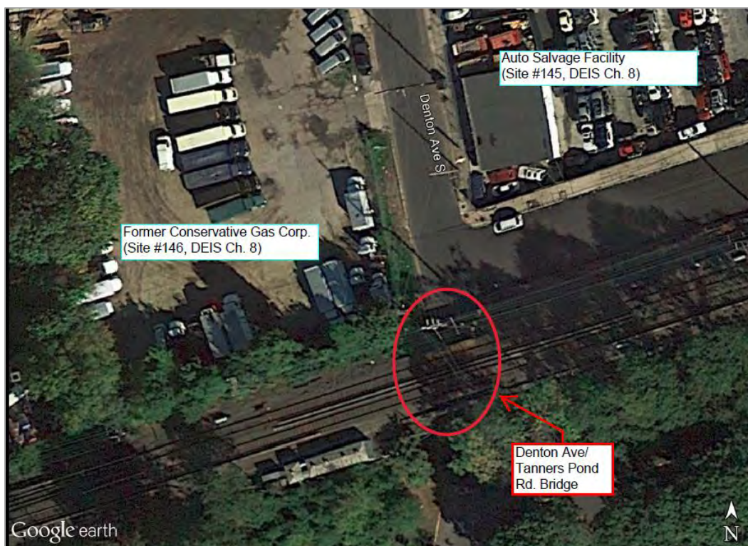
Figure 3.2 – Denton Avenue/Tanners Pond Road Bridge
