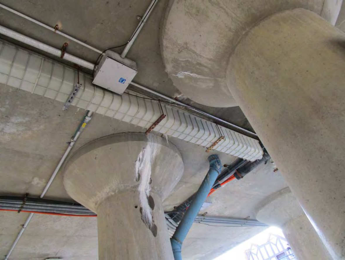
15. & 16. LIRR Commuter Parking Lot Icicles, water dripping from tracks above
