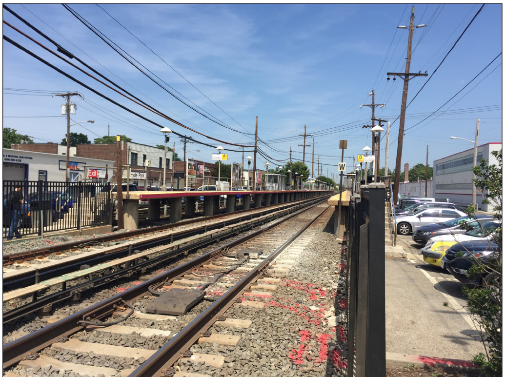
View of railroad tracks at South 12th Street grade crossing, facing northeast. 6
