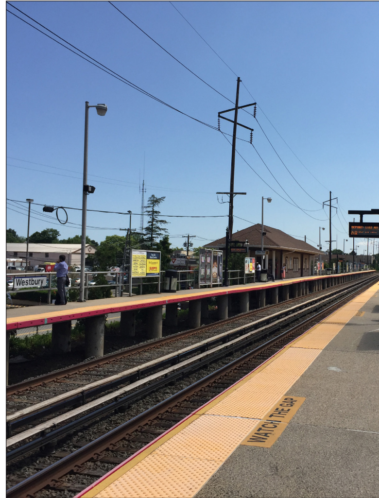
View of railroad tracks at Westbury Station, facing east. 22
