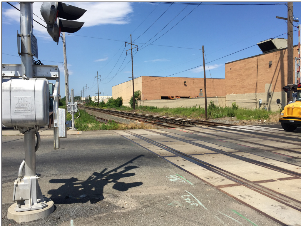
View of grade crossing at School Street, facing west. 23
