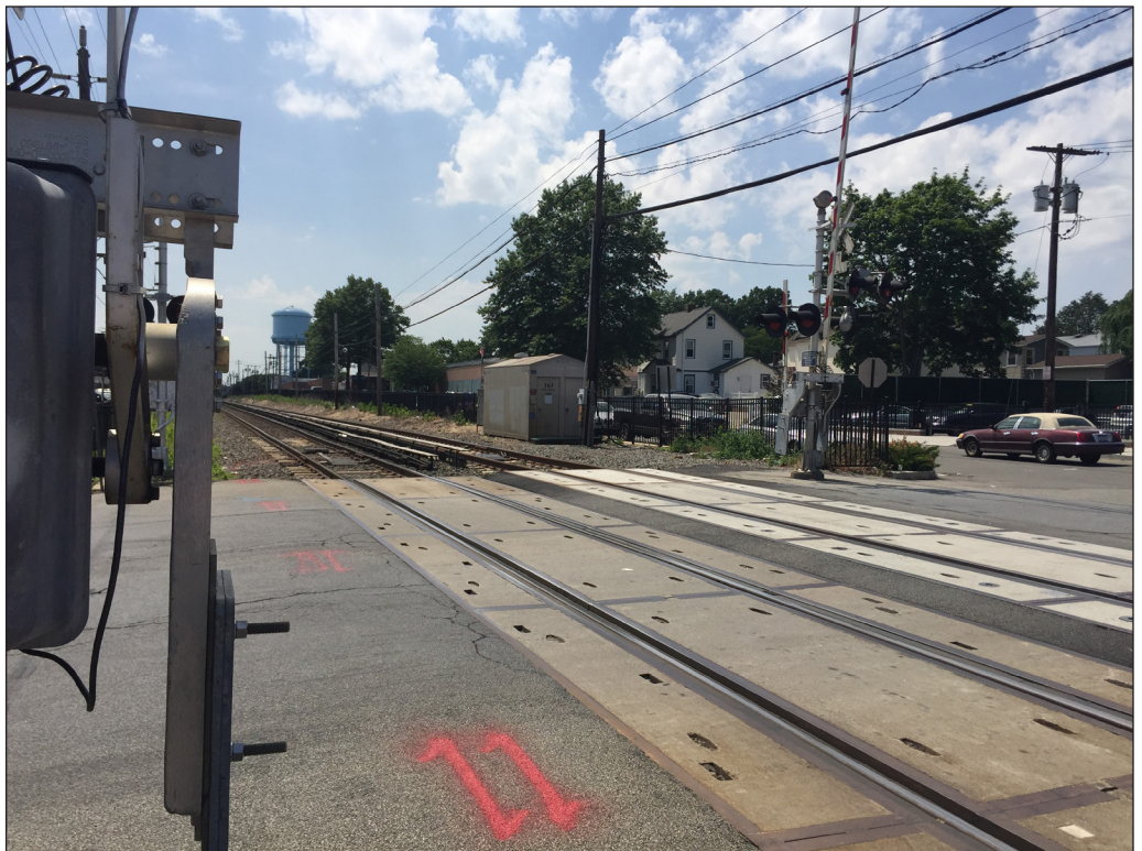
View of grade crossing at South 12th Street, facing northwest. 5
