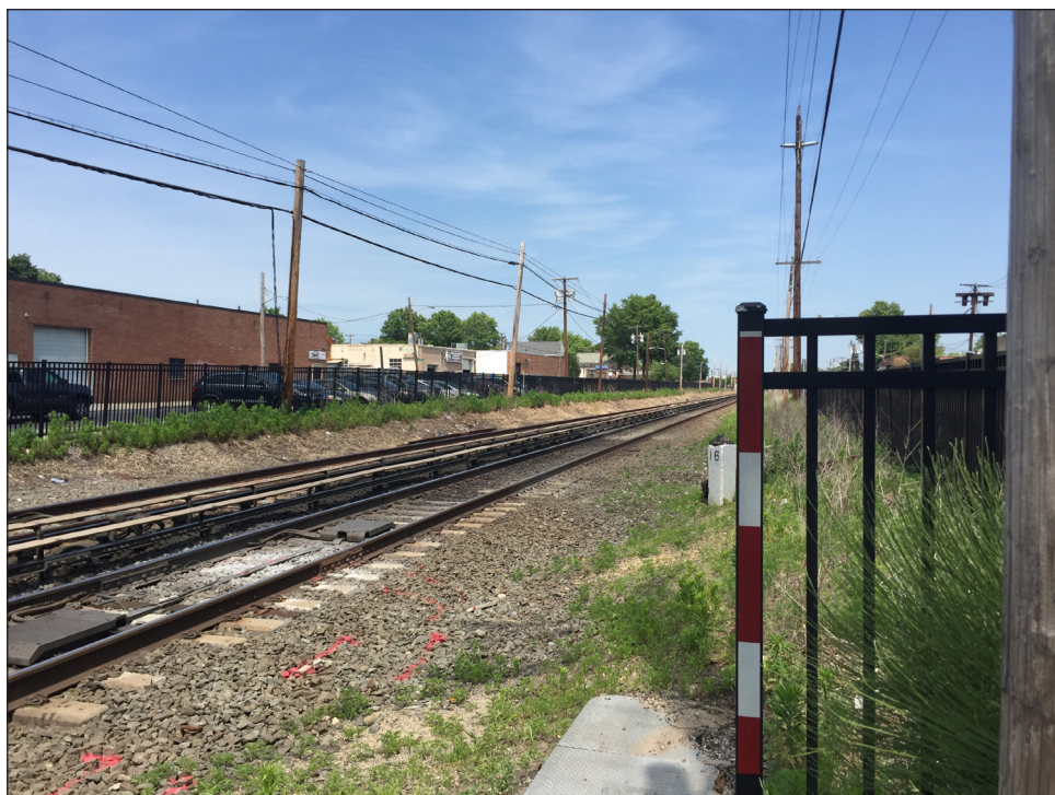
View of railroad tracks at Covert Avenue grade crossing, facing east. 4
