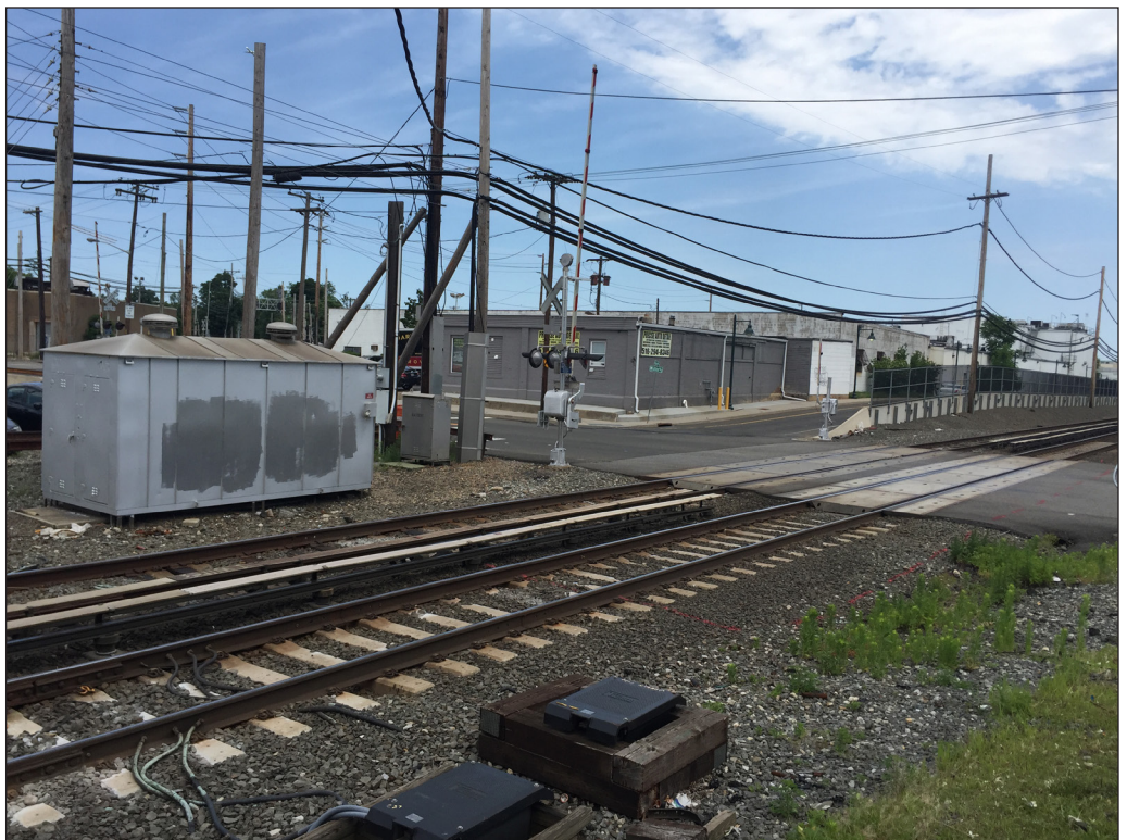
View of grade crossing at Willis Avenue, facing northeast. 18
