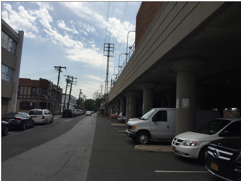
View of Floral Park Station from street, facing west. 1
