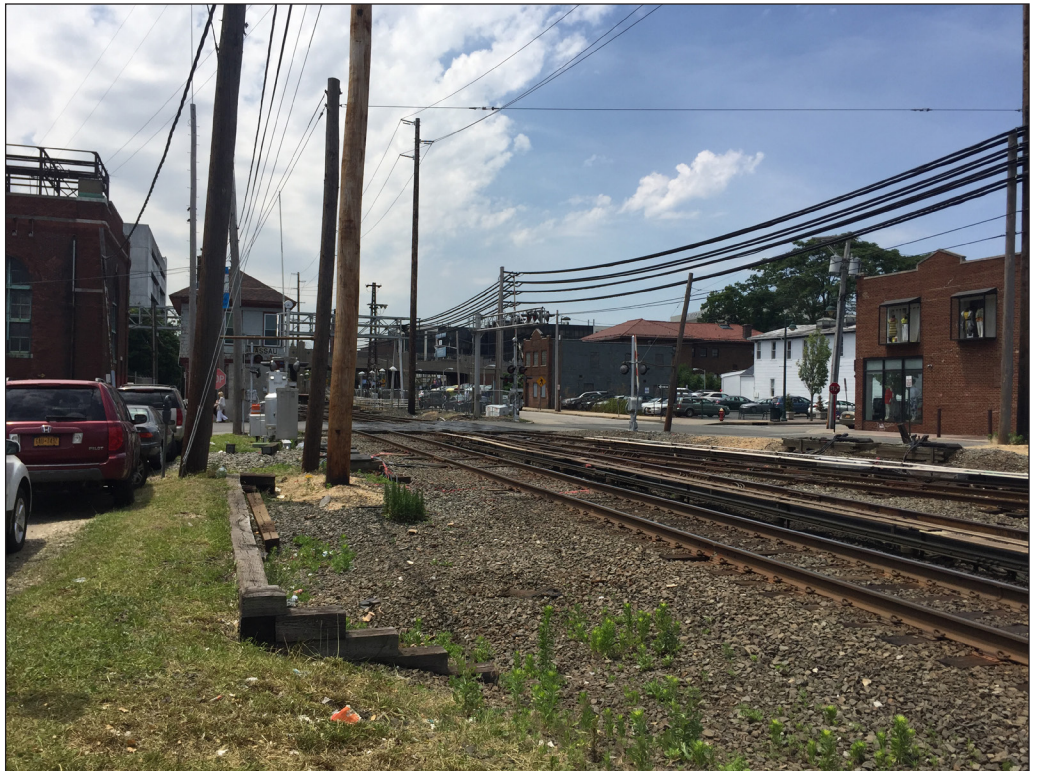
View of grade crossing at Main Street, facing west. 15
