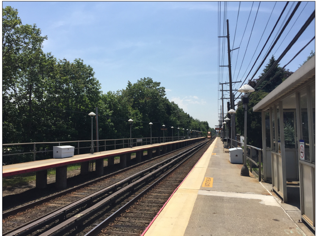
View of railroad tracks at Merillon Avenue Station, facing west. 11
