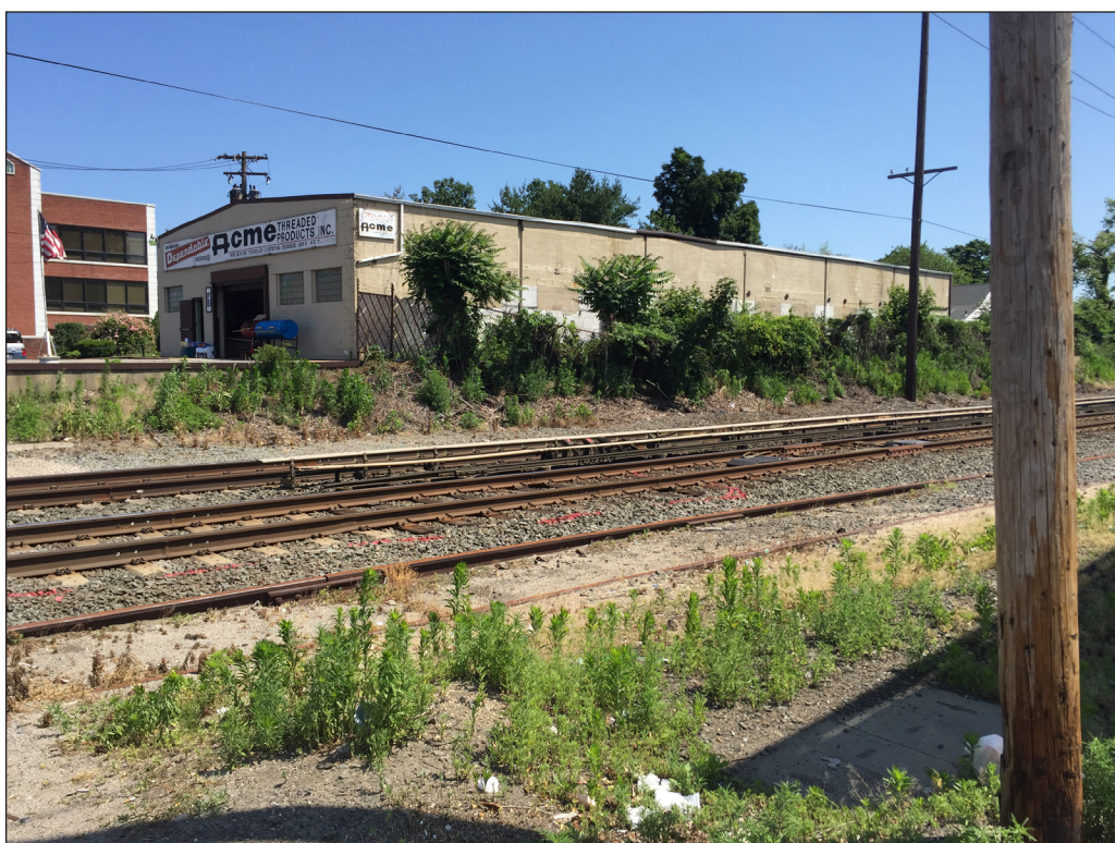
View of railroad tracks at School Street grade crossing, facing northeast. 24
