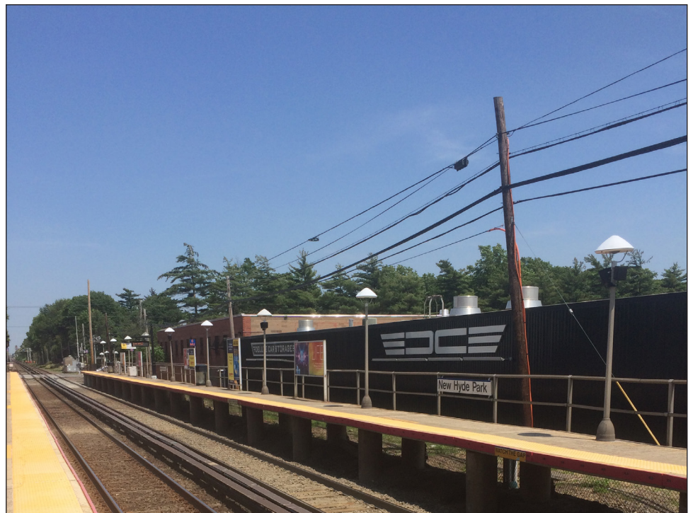
View of railroad tracks at New Hyde Park Station, facing east.
