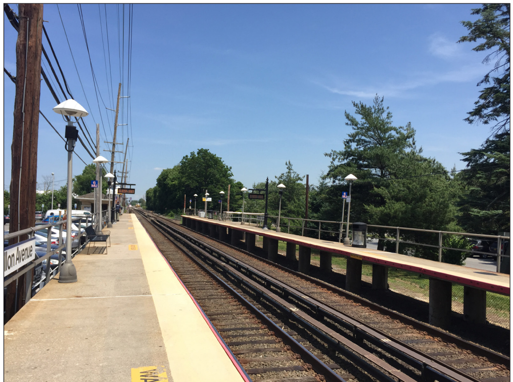
View of railroad tracks at Merillon Avenue Station, facing east. 12
