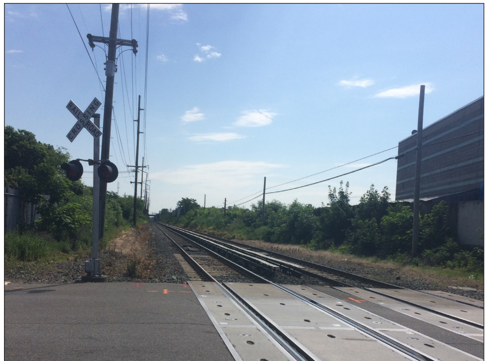
View of grade crossing at Urban Avenue, facing southeast. 26
