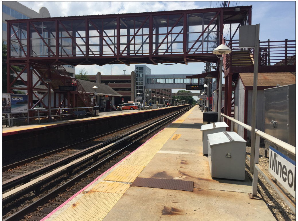
View of railroad tracks at Mineola Station, facing west. 13
