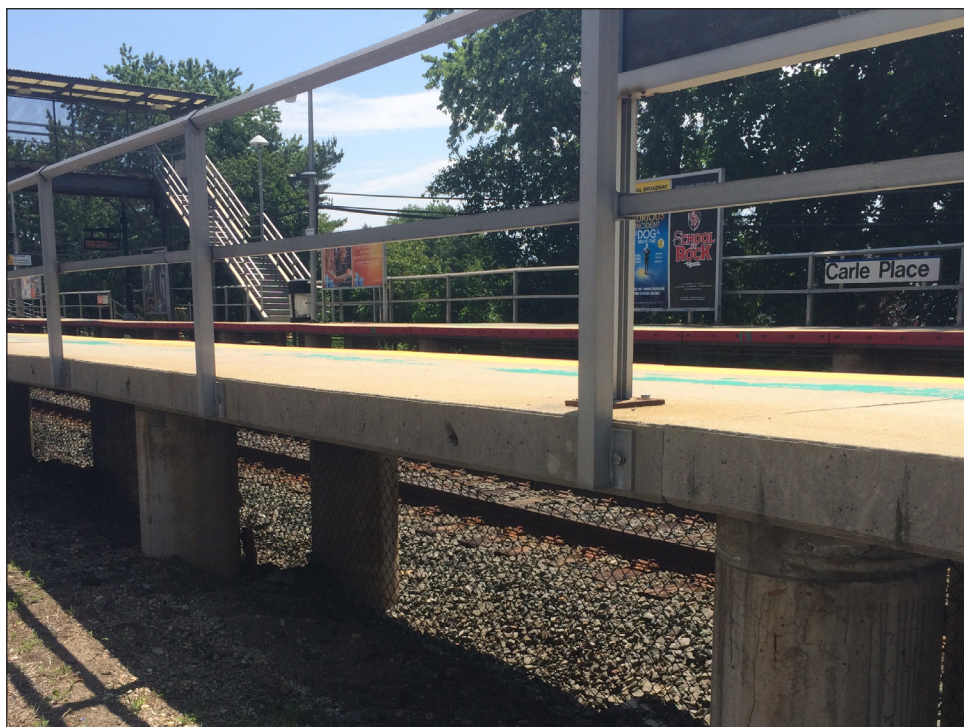
View of Carle Place Station, facing southeast. 20
