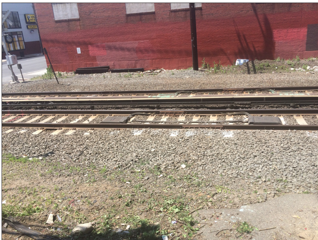
View of railroad tracks at New Hyde Park Road grade crossing, facing north. 10
