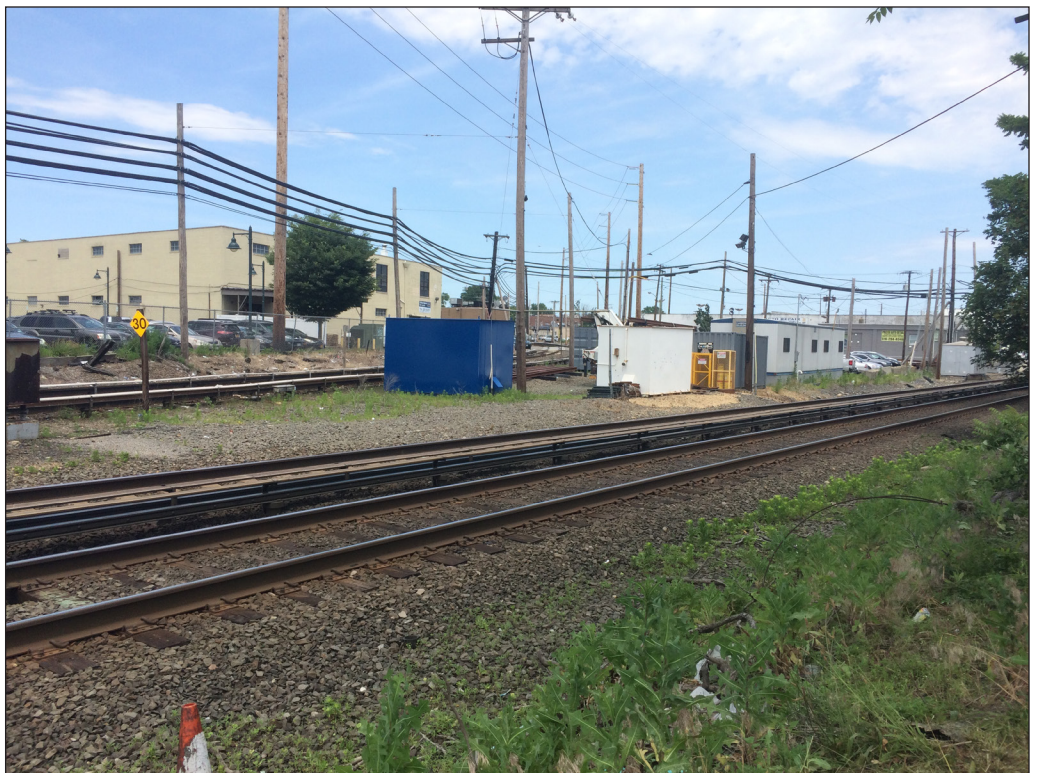
View of railroad tracks at Main Street grade crossing, facing northeast. 16
