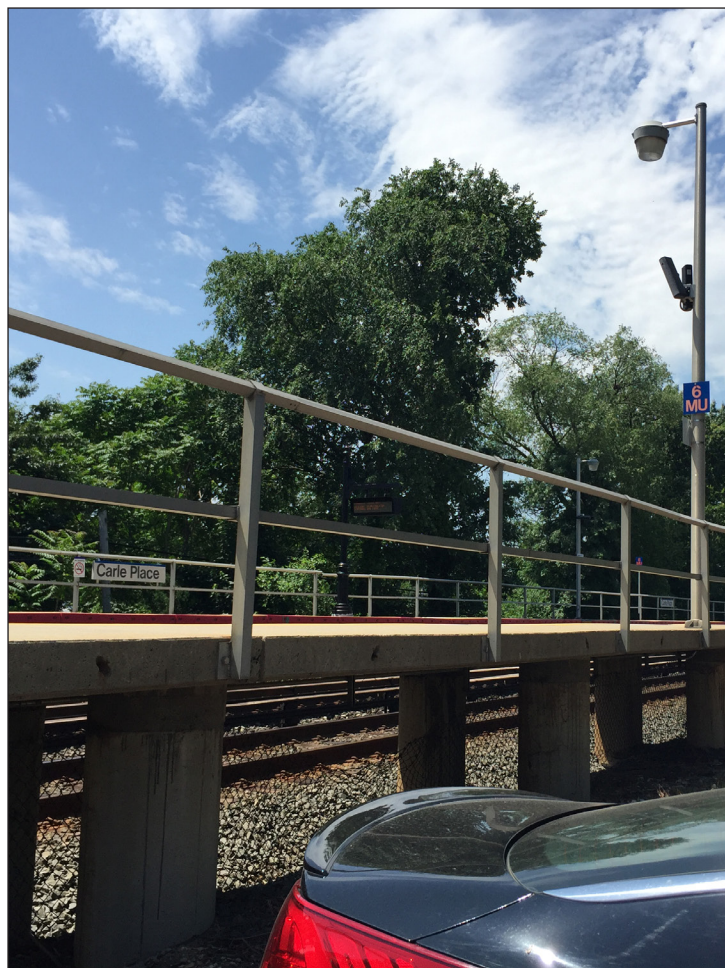
View of Carle Place Station, facing southwest. 19
