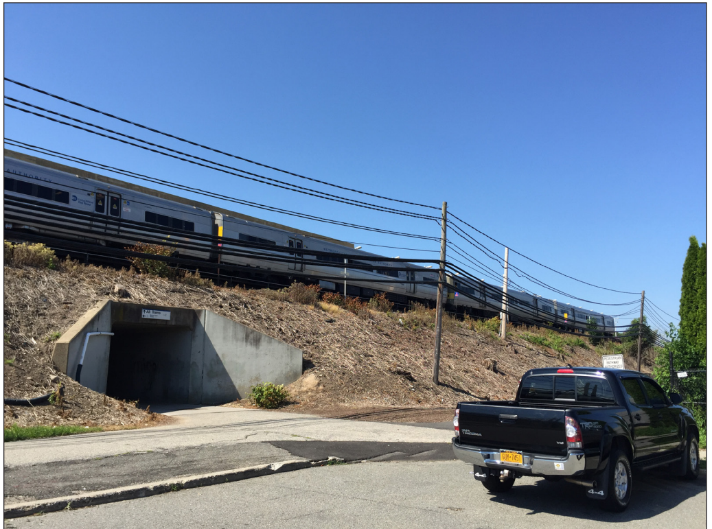
View of Hicksville Station from parking lot, facing southwest. 27
