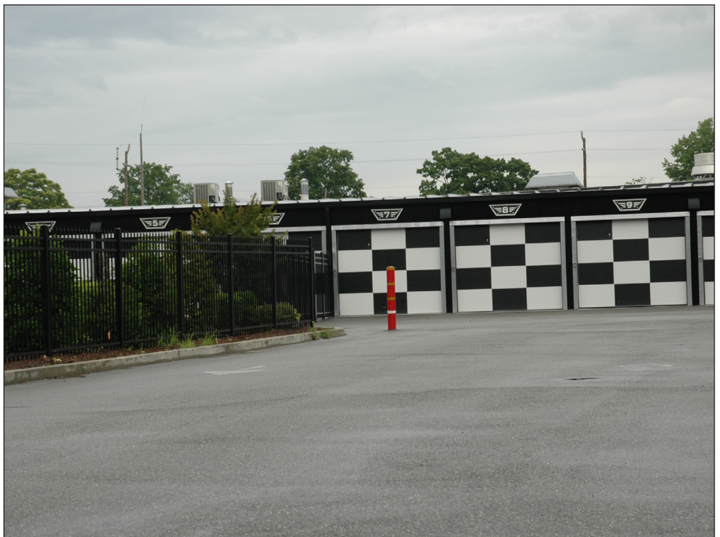
View north towards New Hyde Park Station from 4th Avenue 36
