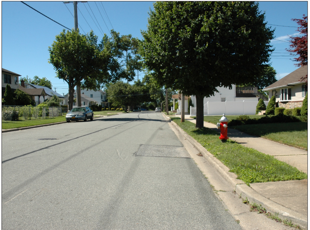
View south from Gardner Avenue onto Project Corridor 171
