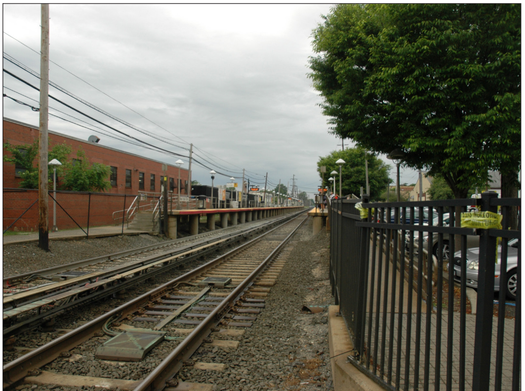
View west from New Hyde Park Road Grade Crossing towards New Hyde Park Station 40
