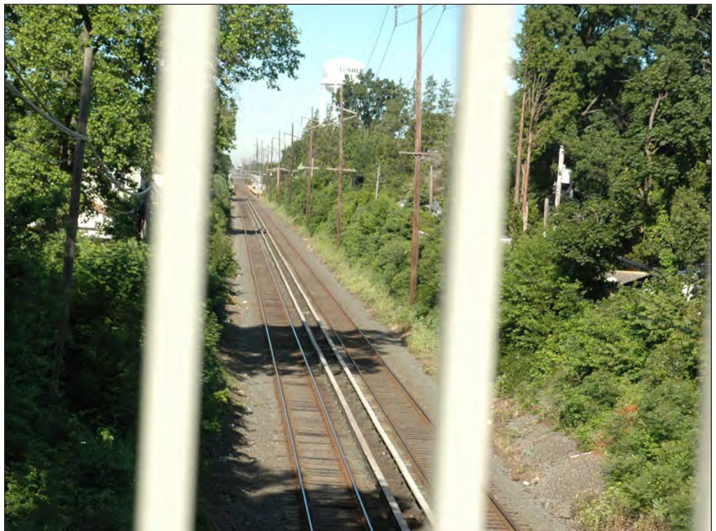
View west from Ellison Avenue Bridge onto Project Corridor 120
