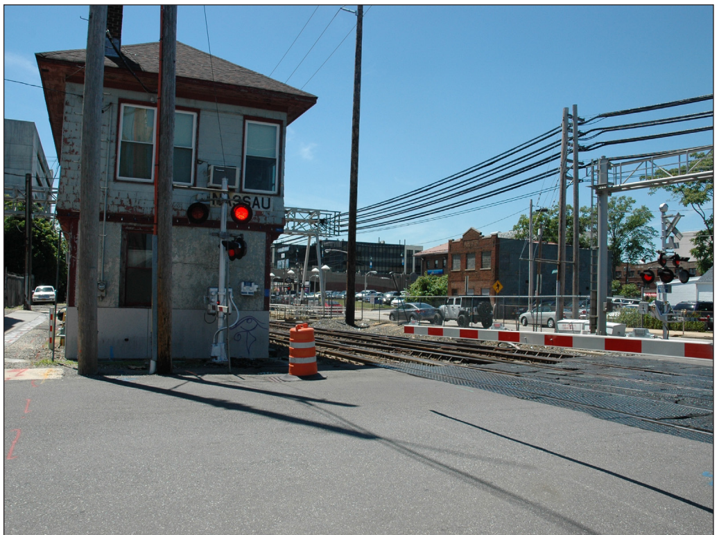
View northwest from Main Street towards Main Street Grade Crossing 82
