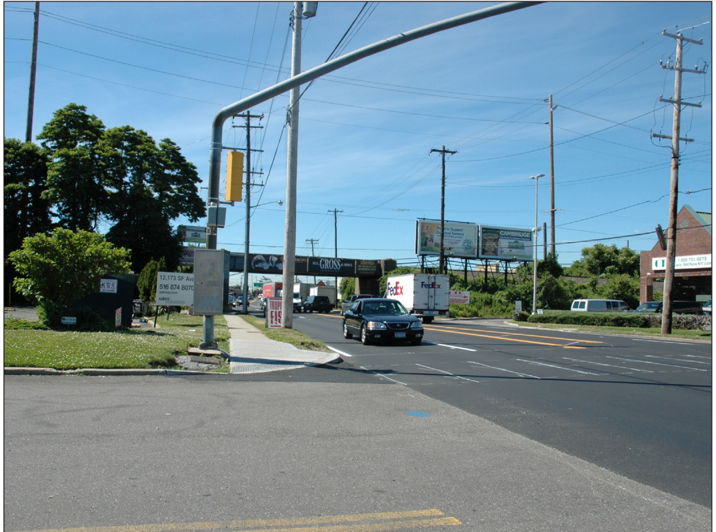
View south towards Glen Cove Road towards Glen Cove Road Bridge Crossing 106
