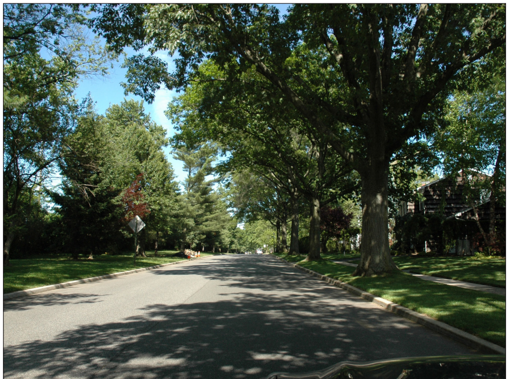
View west towards Project Corridor from Main Avenue 50
