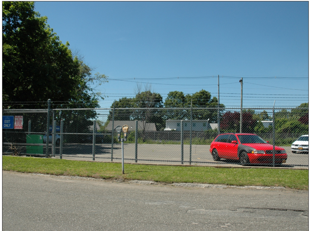
View north onto the Project Corridor from 8th Avenue 69
