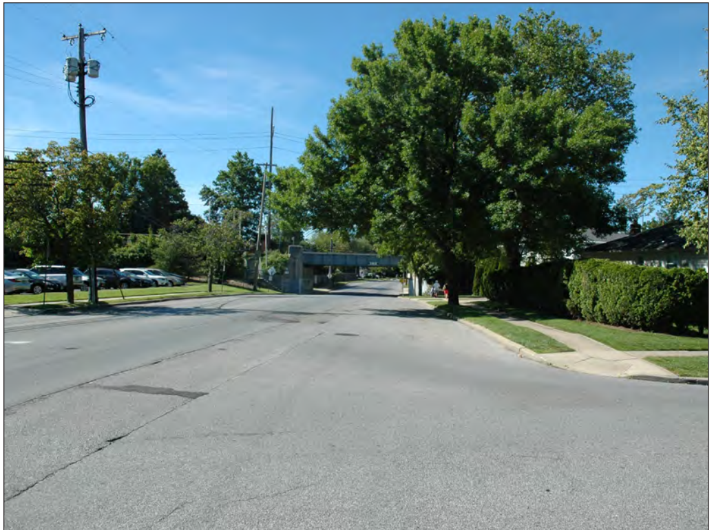
View south from Cherry Lane towards Cherry lane Bridge Crossing 111
