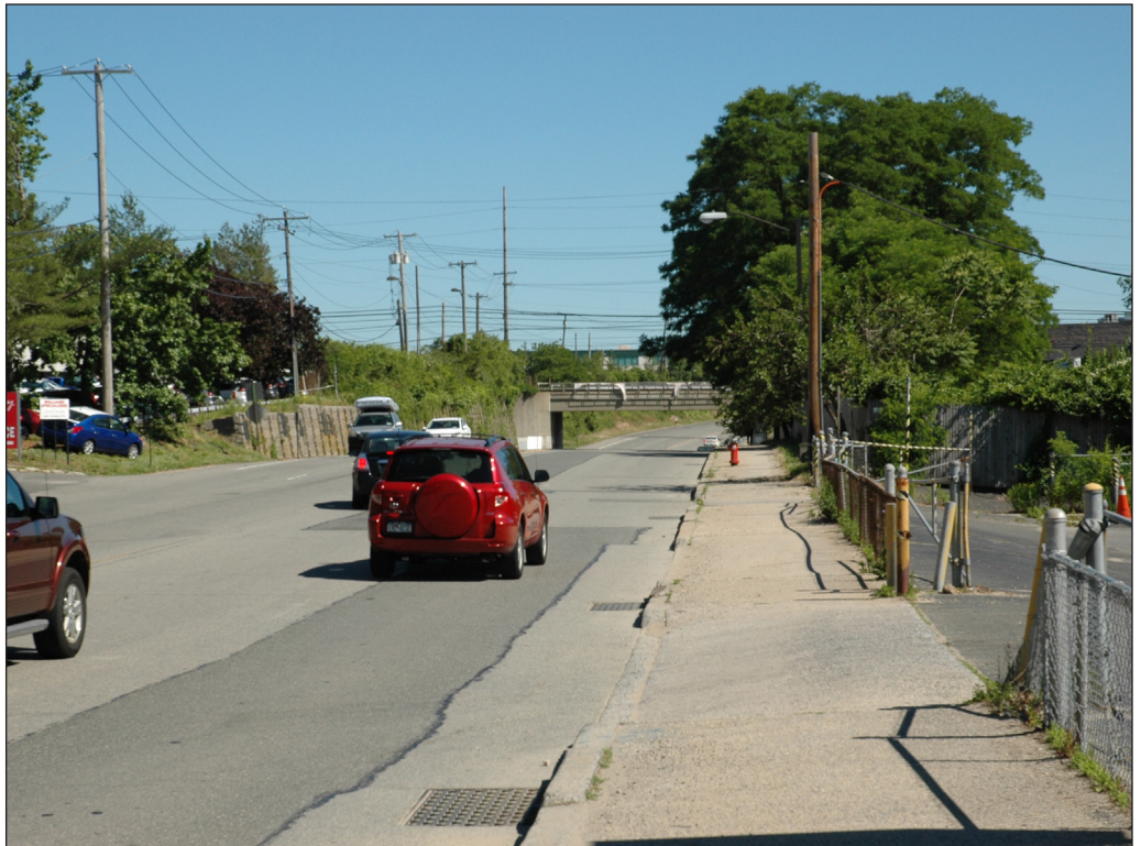
View south from Charlotte Avenue onto Charlotte Avenue Project Corridor 173
