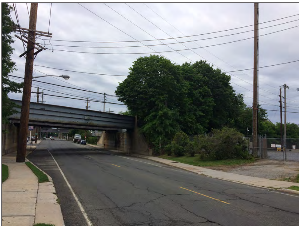
View south towards Project Corridor from Plainfield Avenue 10
