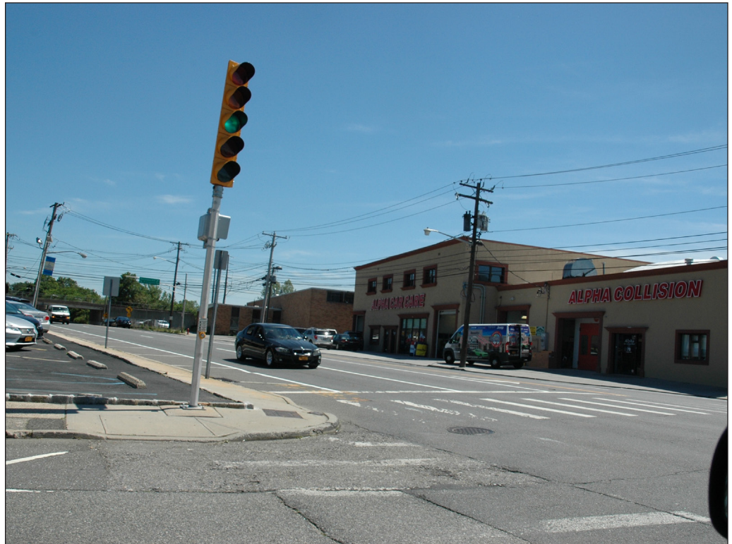
View south onto Herricks Road Bridge Crossing 65
