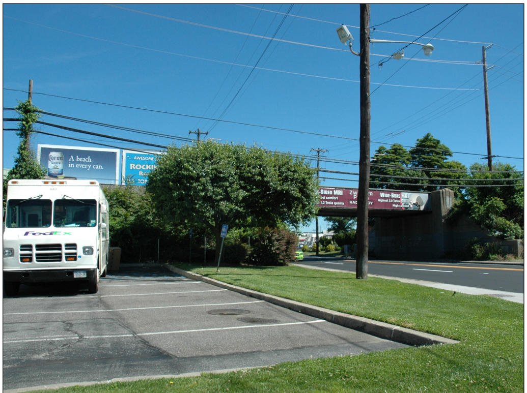
View north from Glen Cove Road towards Glen Cove Road Bridge Crossing 107
