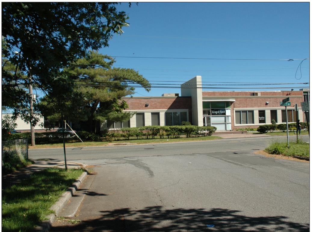
View north from Loretta Lane towards Project Corridor 176
