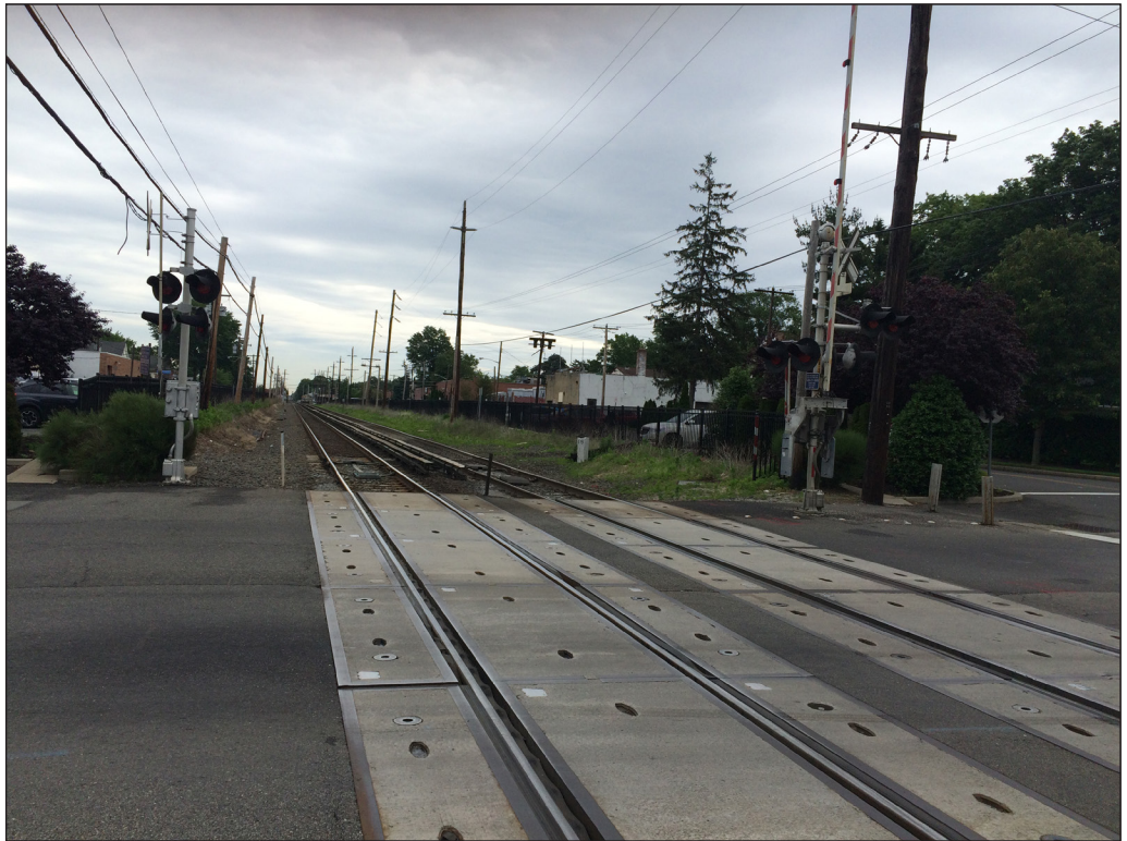
View west towards Project Corridor from Second Avenue and Covert Avenue 22
