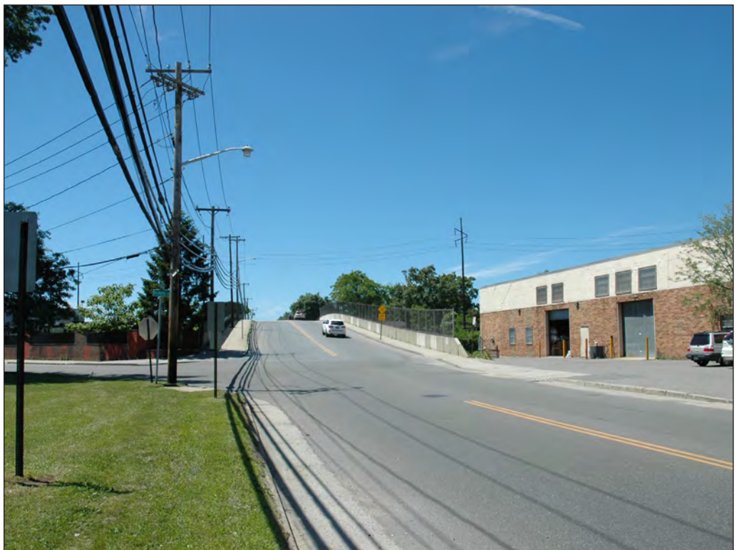
View north from Grand Street Boulevard towards Grand Street Bridge Crossing 146
