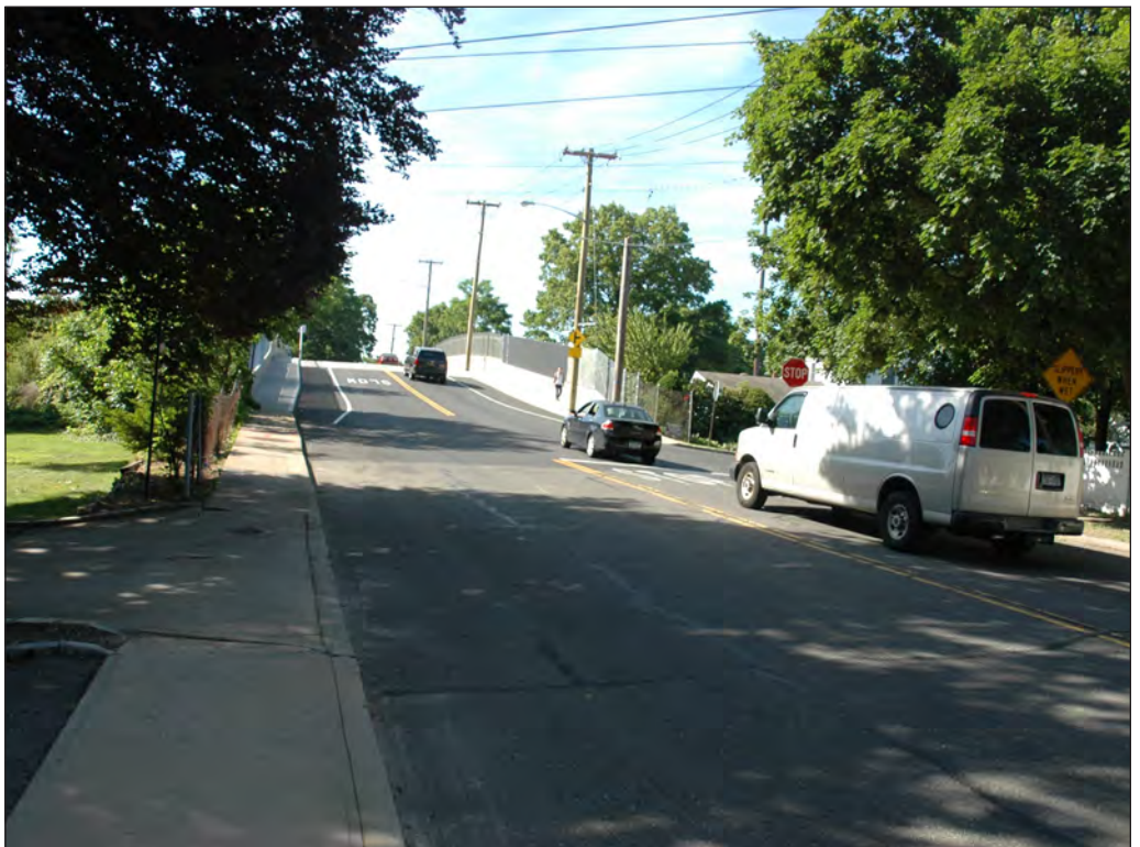
View south from Ellison Avenue towards Ellison Avenue Bridge Crossing 118
