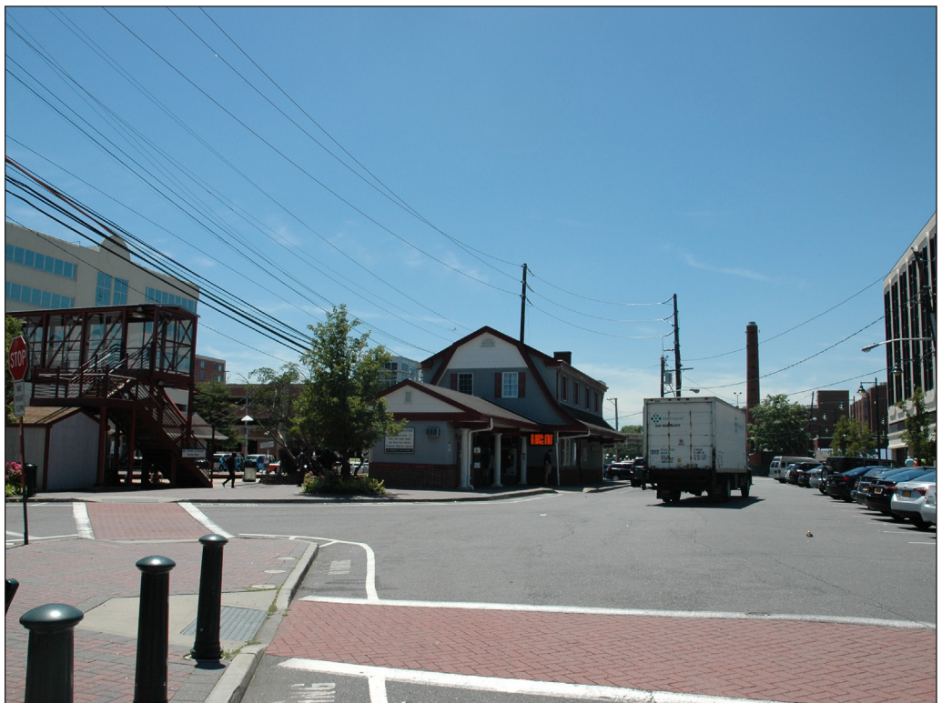
View southwest onto Mineola Station 76
