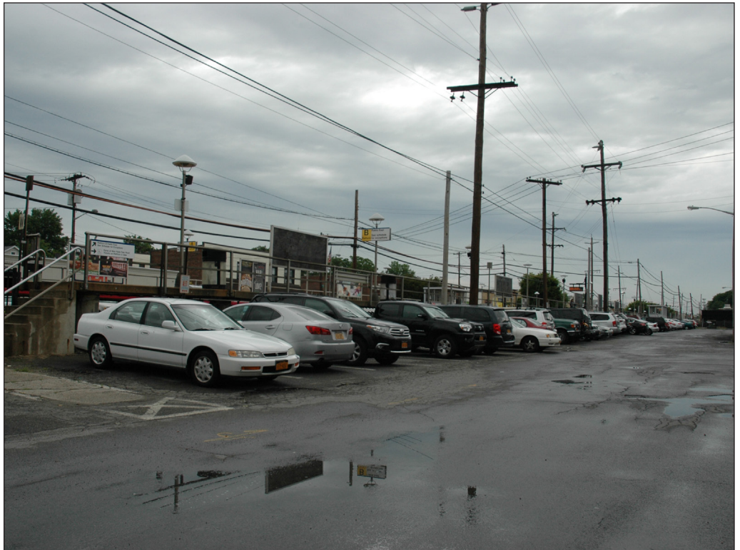
View east towards New Hyde Park Station 35
