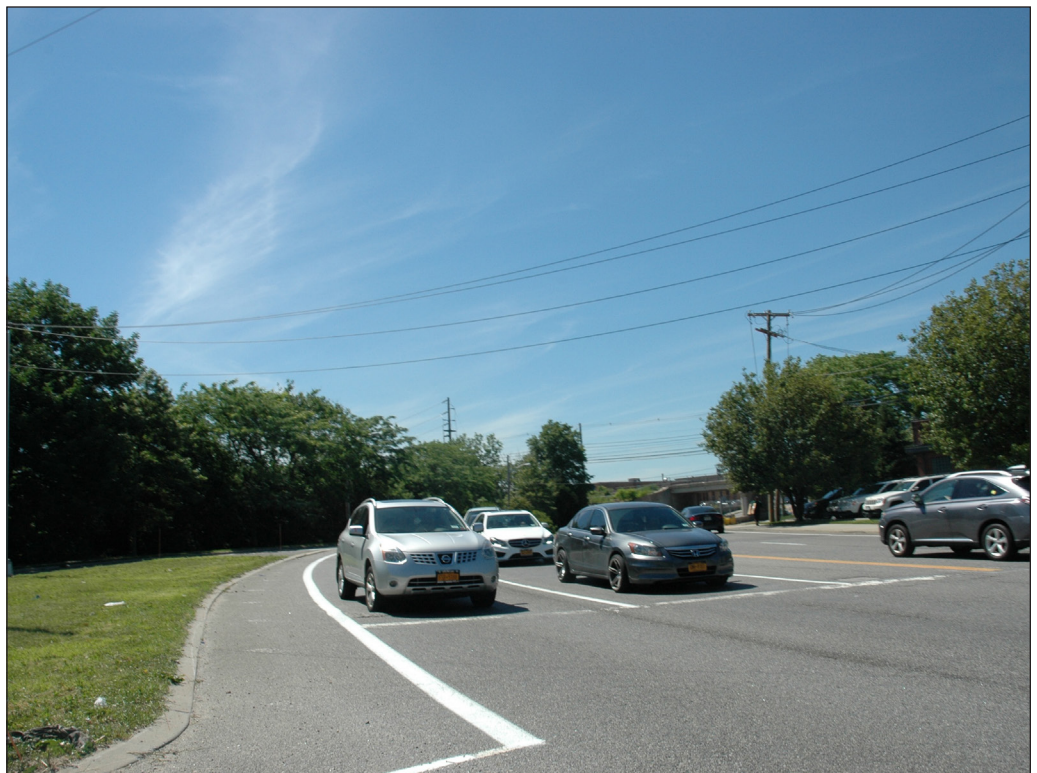
View north onto Herricks Road Bridge Crossing 64
