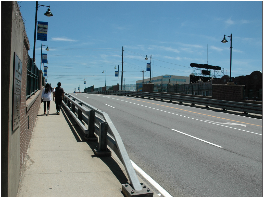
View south onto Franklin Avenue Bridge Crossing 78
