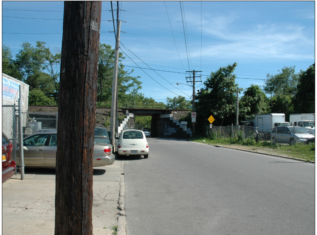
View south towards Tanners Pond Road/Denton Avenue South Bridge Crossing 49
