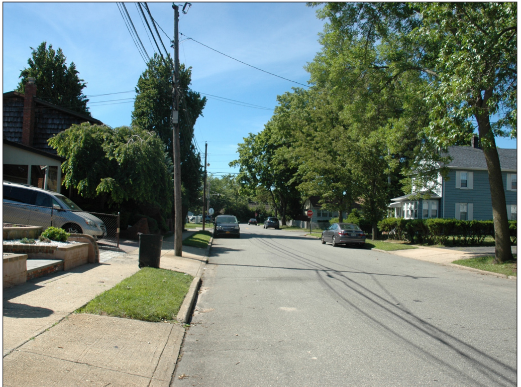
View south from Silver Lane towards Project Corridor 108
