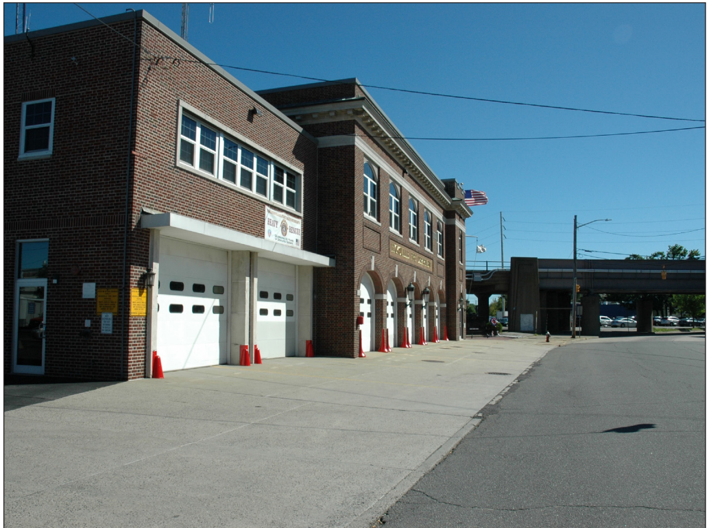
View north from Hicksville Volunteer Fire Department towards Project Corridor 178
