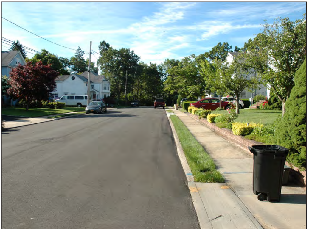
View south from Manor Avenue towards Project Corridor 126
