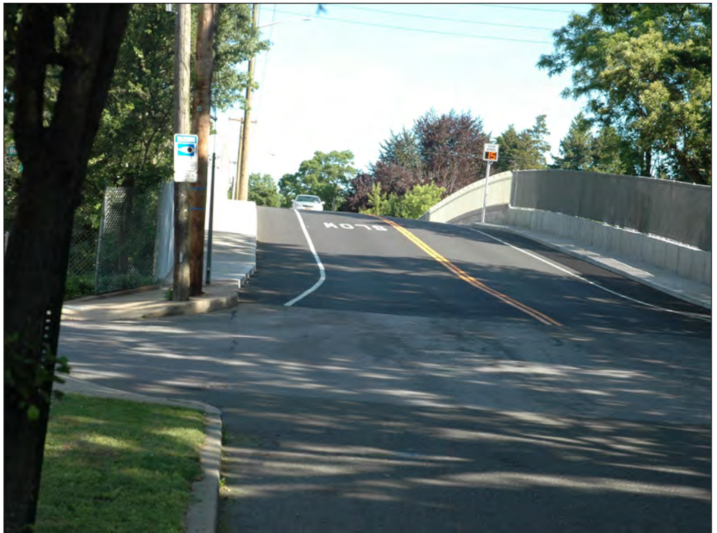
View north from Ellison Avenue towards Ellison Avenue Bridge Crossing 121
