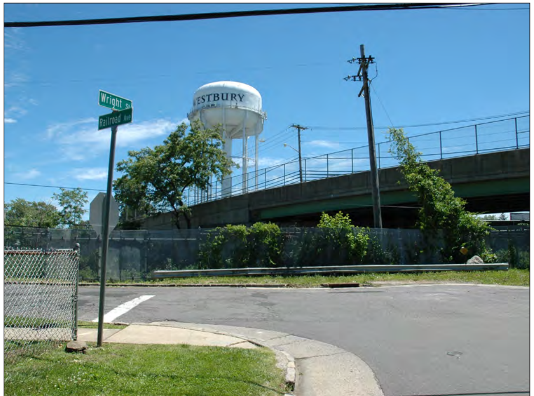
View south from Wright Street towards Project Corridor 149
