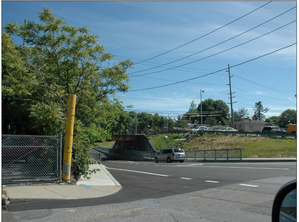
View south towards Nassau Boulevard Bridge Crossing from Nassau Boulevard 55
