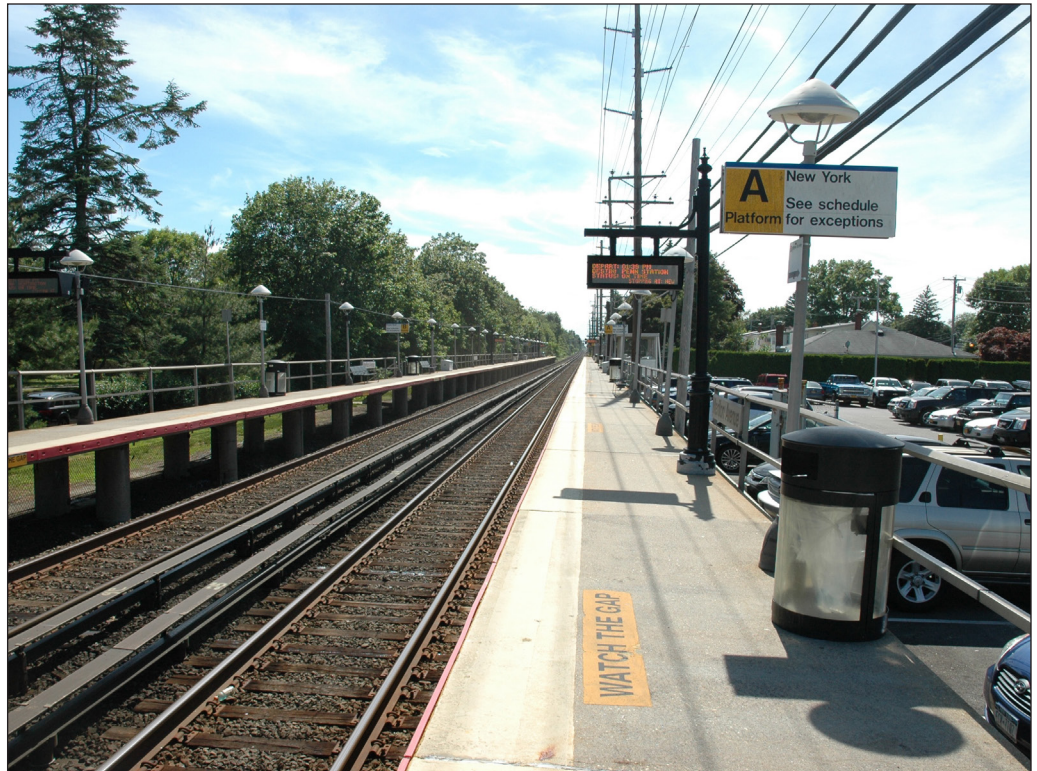
View west from Merillon Avenue Station 53
