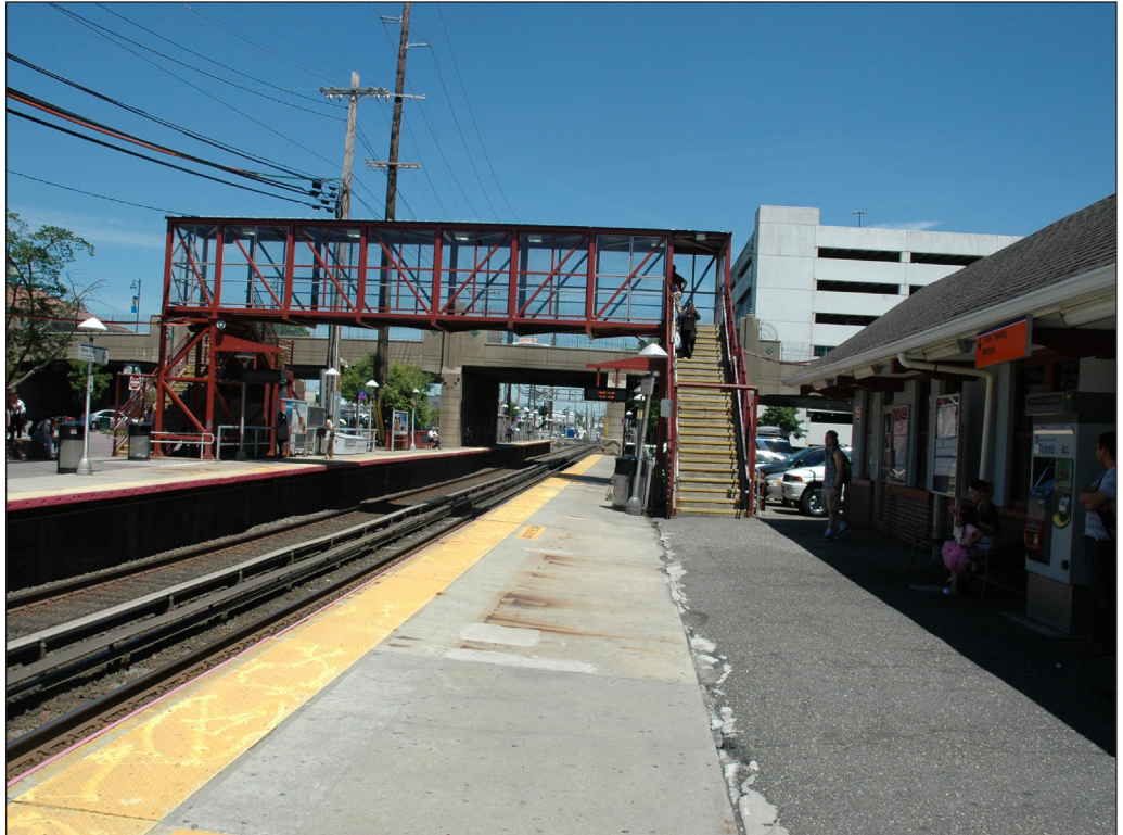
View east from Mineola Station 75
