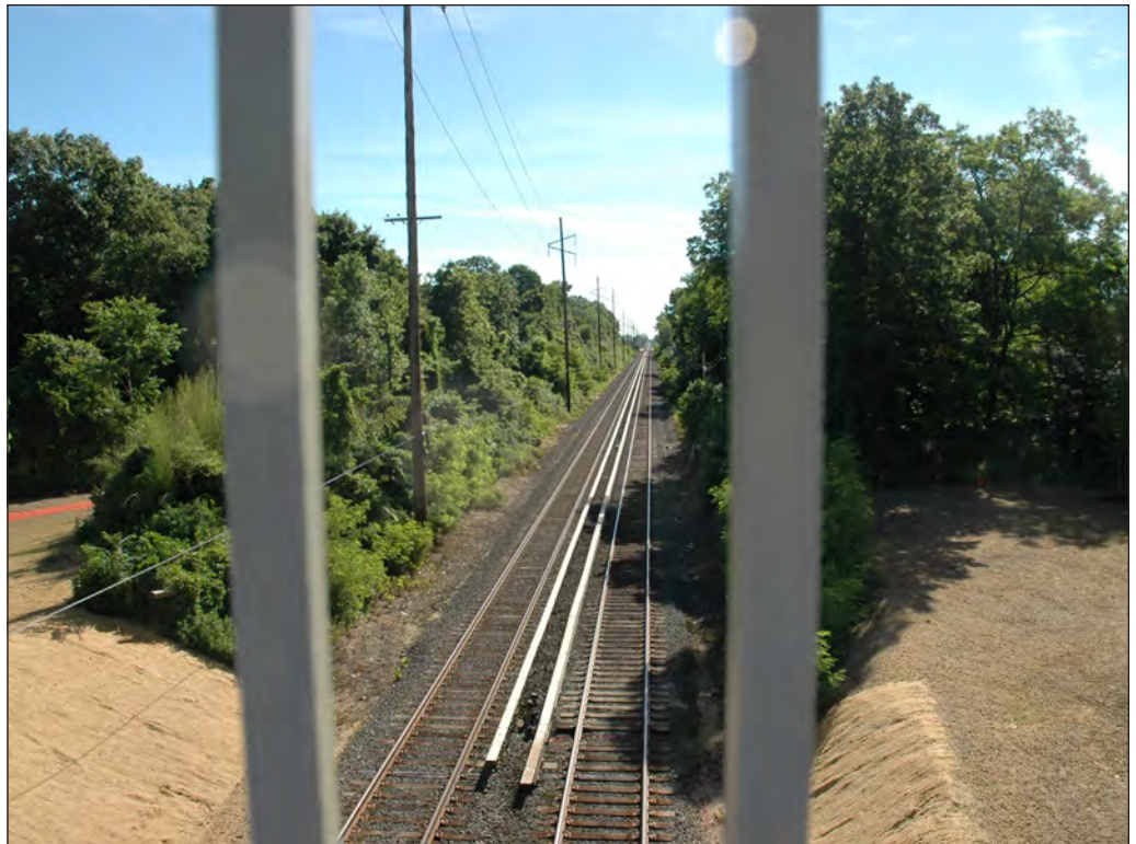
View east from Ellison Avenue Bridge onto Project Corridor 119
