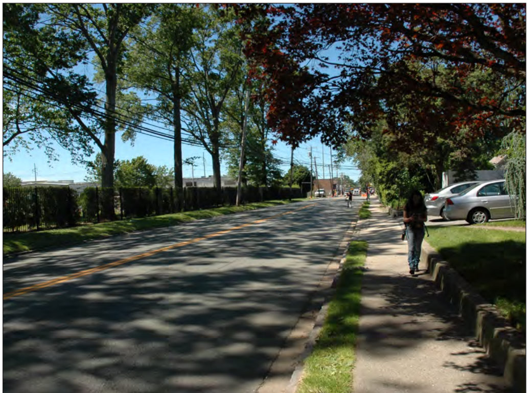
View east from Railroad Avenue towards School Street Grade Crossing 142
